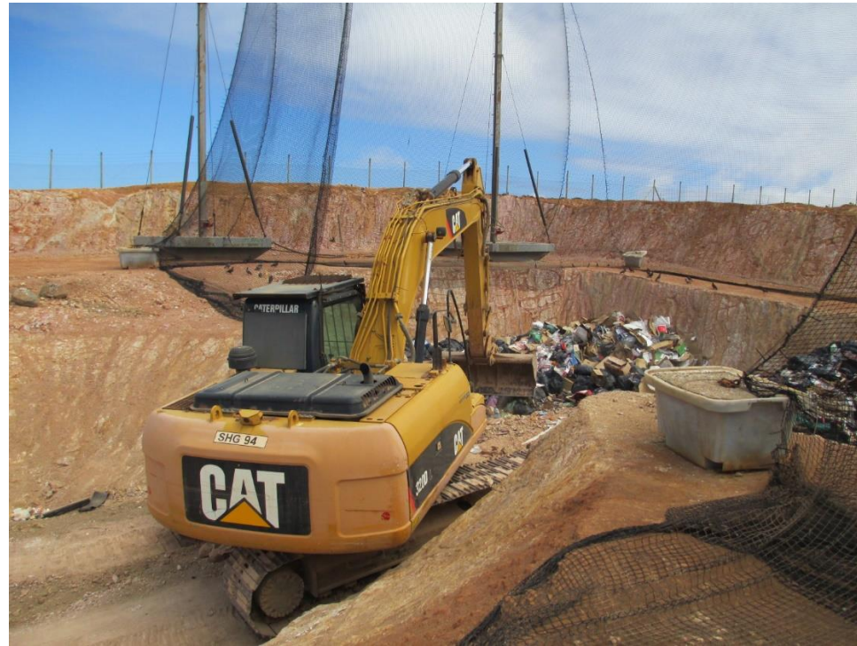
CAT Excavator landfilling waste at Horse Point Landfill Site
