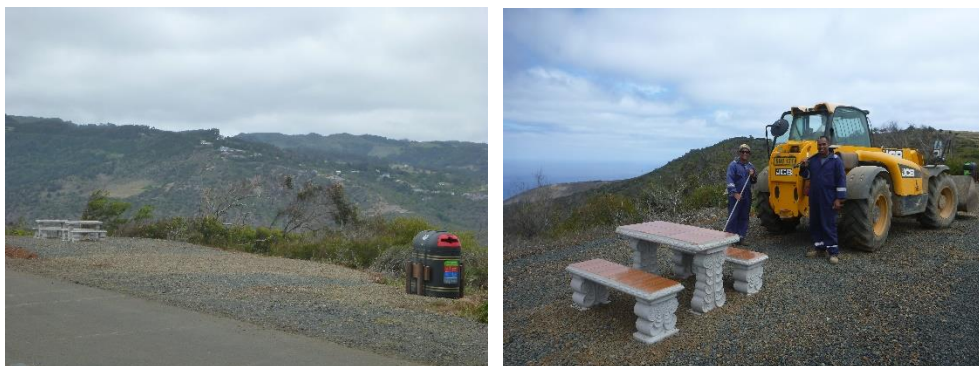
Public space along the Access Road near Deadwood – designed and delivered by Waste Management Services – 2019
