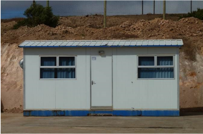
2.9 New site office at HPLS, Jun 16
