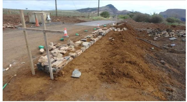
2.2 Re-construction of a section of the Great Wood Wall, Aug 16
