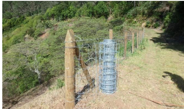
2.6 Fencing at Peak Dale compensatory site, Jan 17
