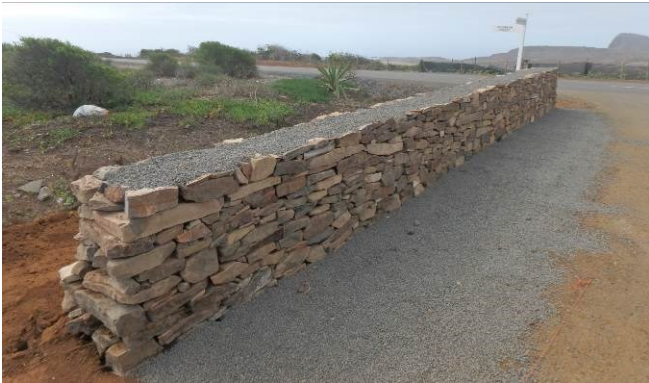
2.3 Completed section of the Great Wood Wall, Aug 16
