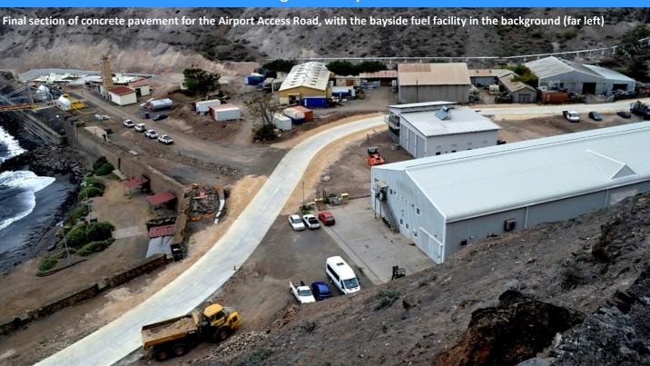
Airport Project works in Rupert's continue, with the recent completion of the concrete road section from the Wharf to the Basil Read workshop site (the building previously used as the Cannery). Works will now focus on the installation of electricity and water services to the Wharf.
