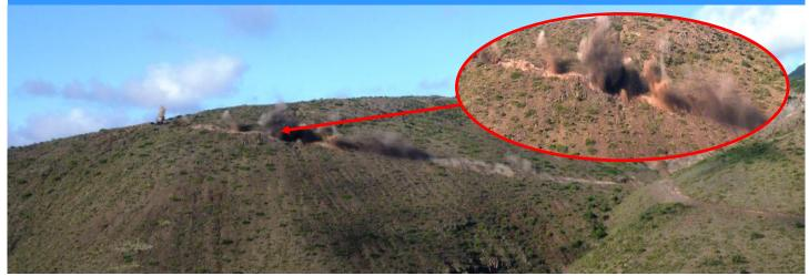
Blasting on the Haul Road in upper Rupert's Valley took place on Tuesday 11 March 2014 just after 5pm. The main purpose of the blast was to assist the heavy plant to excavate the harder section of the track to improve the widths and the gradients to form an Access Road for ultimate public use in the future. 8,513kg of high energy fuel (explosives) was used in the blast - it lasted 5.78 seconds and produced 17,881m³ (approx 34,000 tonnes) of material.
