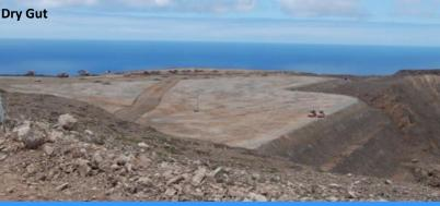
Earlier this month the Dry Gut fill reached 270m in height. The filling of Dry Gut is required to extend the platform available for construction of the runway and the runway end safety areas.
