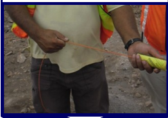
2. Charges inserted into holes
