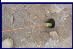
3. A network of charging leads form a grid
