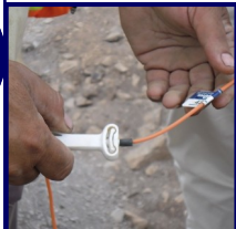
6. Detonator charged and placed within explosive holes.
