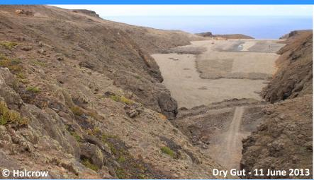
Last week saw the 100,000th truckload of fill going into Dry Gut. This is equivalent to nearly 19% of the total required.
