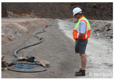
Basil Read are installing settlement monitors which will monitor the fill in Dry Gut during the construction period and enable assessment of the creep settlement after construction. The system consists of a series of differential settlement monitoring gauges connected by a fluid filled hydraulic line at intervals through the fill.
