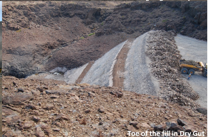
Water added to fill material before going into Dry Gut
