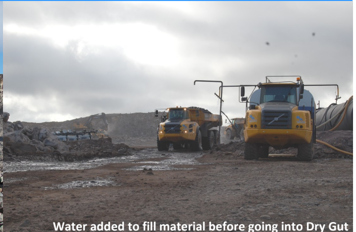
Water added to fill material before going into Dry Gut
