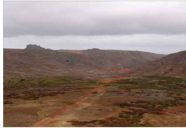
Photo 106: Section 4 Water Pipeline
