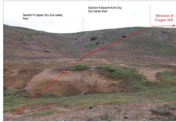
Photo 107: Section 5 Water Pipeline
