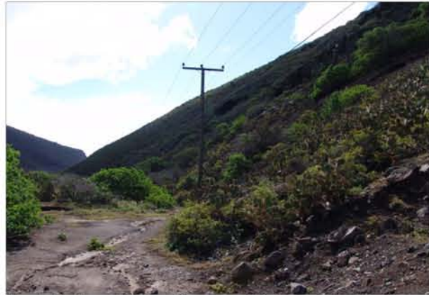
Photo 9: Upper Valley Proposed Bulk Fuel Installation
