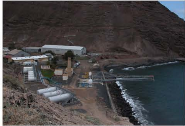
Photo 5.5: Existing Bulk Fuel Installation at Rupert's Bay
