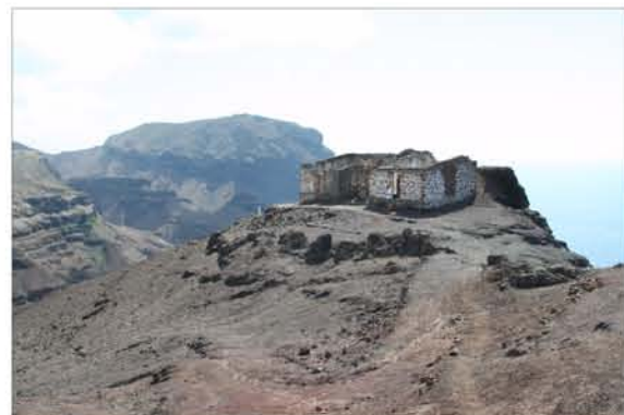
Photo 6.6: The remains of Prosperous Bay Signal Station
