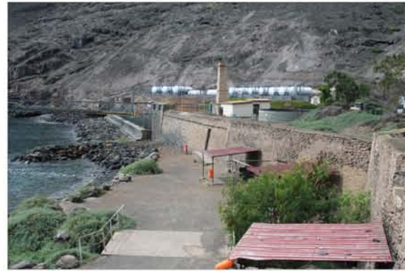
Photo 1.2: Rupert's beach with the bulk fuel farm and desalination chimney beyond
