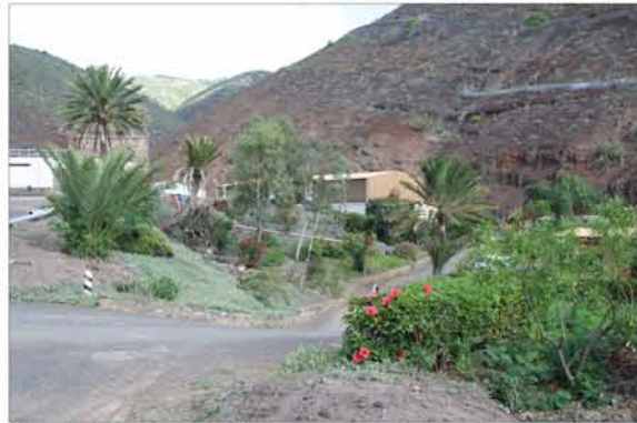
Photo 1.5: Power station and amenity planting
