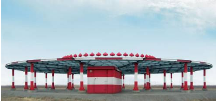
Plate 2.3 Typical DVOR Array
