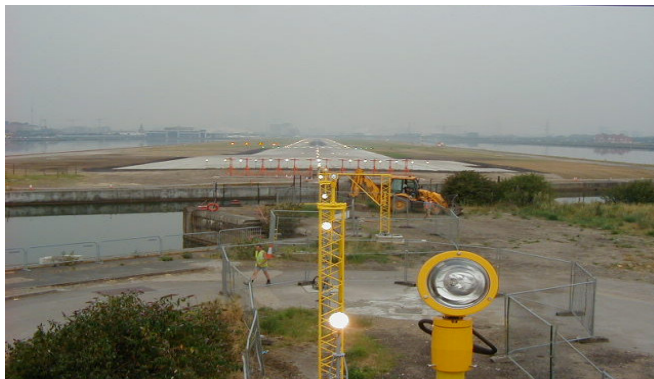
Plate 2.2 Typical Airfield Approach Lighting Structures
