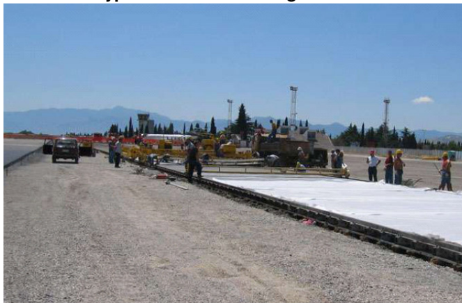
Plate 2.10 - Typical Concrete Paving Machine
