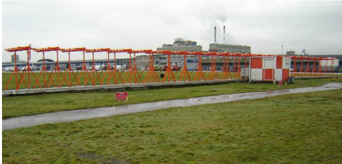
Plate 2.4 Typical Instrument Landing System
