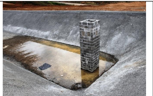
Plate 36: Completed hazardous waste cell with gas release chimney
