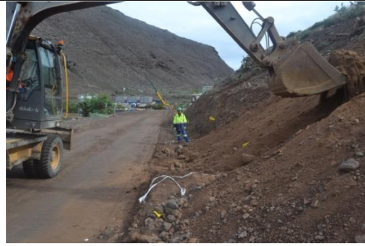
Plate 8: Excavation using a toothless excavator
