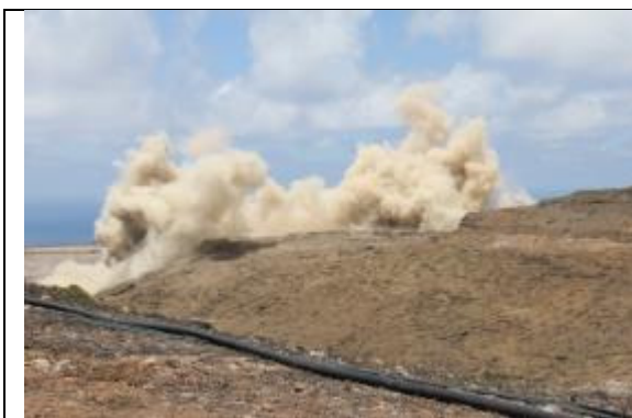
Plate 28: Blasting for the open channel (February 2014)
