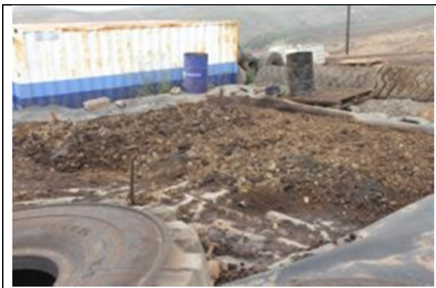
Plate 32: Bioremediation pad in operation at Bradley's. A photo-ionising detector is used to determine when the hydrocarbons have been broken down enough to render the soil as 'clean'.
