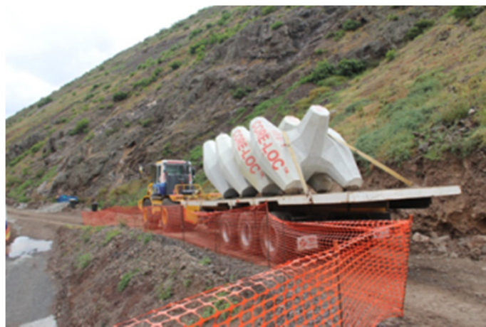
Plate 17: Core-locs being transported from the pre-cast yard in Upper Rupert's Valley to the wharf site
