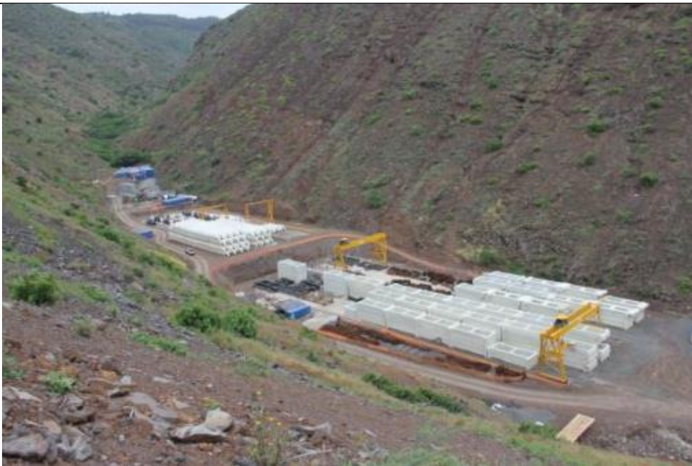
Plate 18: From left to right: concrete batch plant, Core-loc yard and block wall pre-cast yard in upper Rupert's Valley
