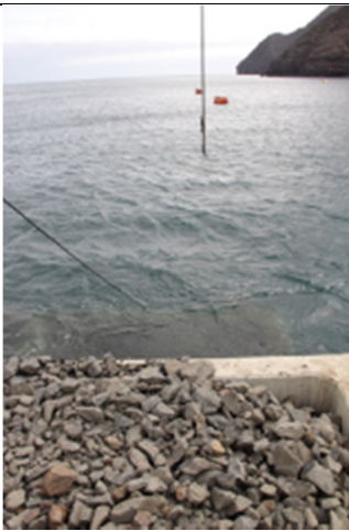
Plate 16: A block wall being filled with crushed rock
