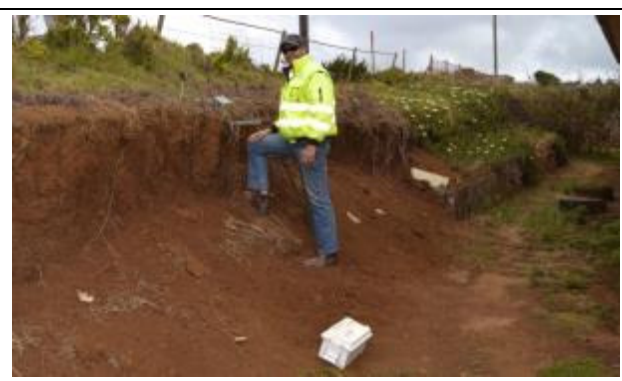
Plate 29: Monitoring vibration during use of the heavy roller near a house in Deadwood (November 2013)
