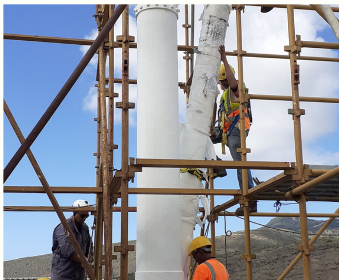
Positioning the flagpole section through scaffolding
