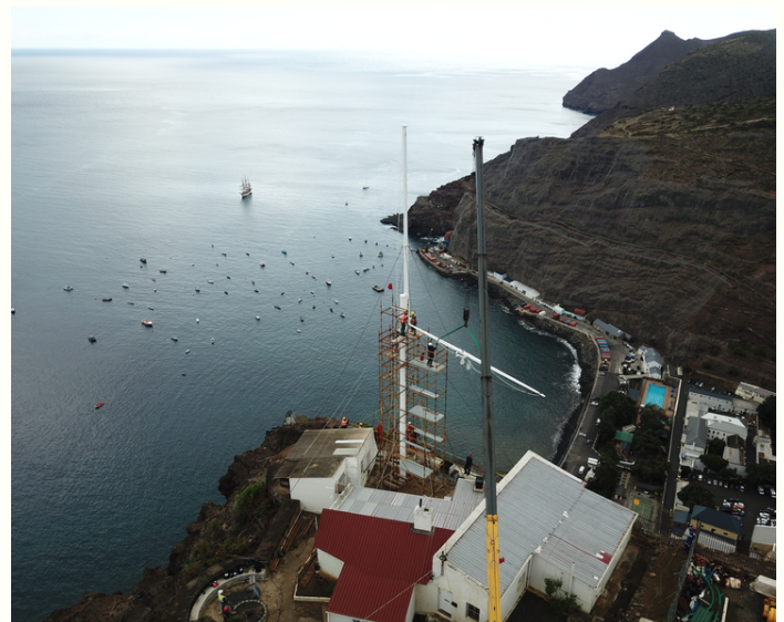
Crane lifting the yard arm
