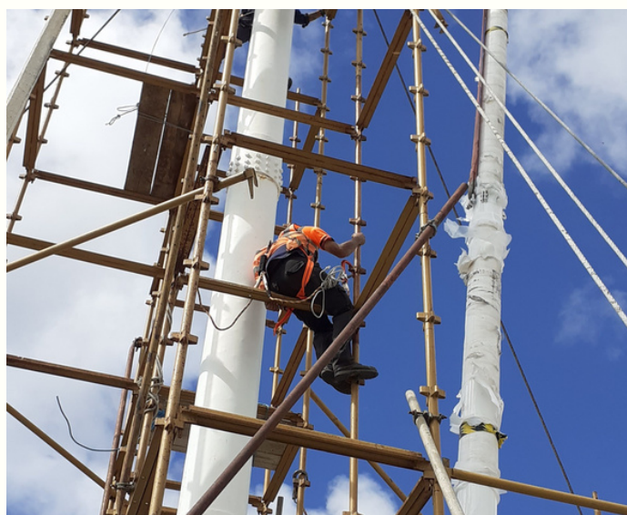
Positioning the flagpole section in place
