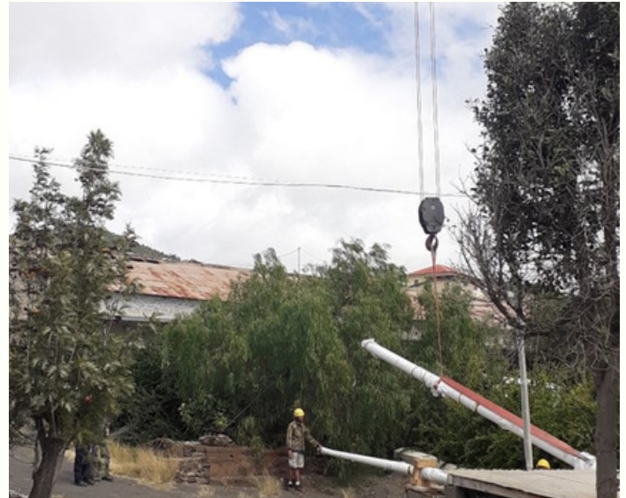
Initial lifting of the flagpole section
