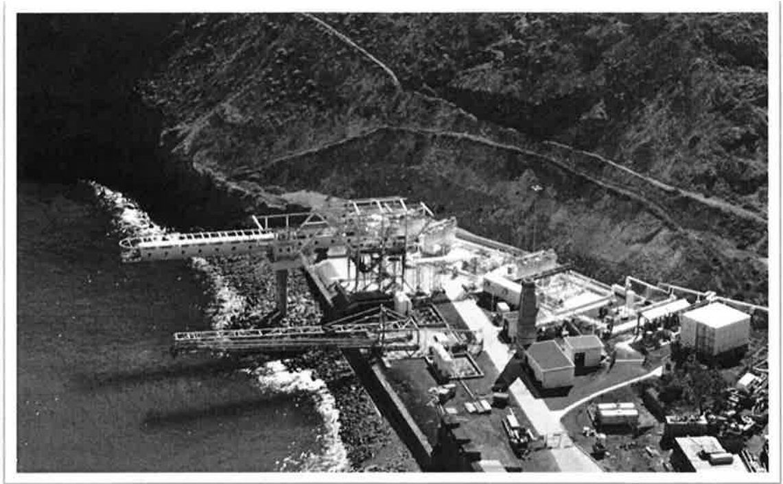
FIGURE 5. BAY SIDE FACILITY INCLUDING OLD AND NEW FUEL GANTRIES, OCTOBER 2019
