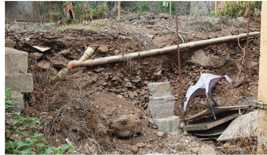
Excavated bank in 2024
