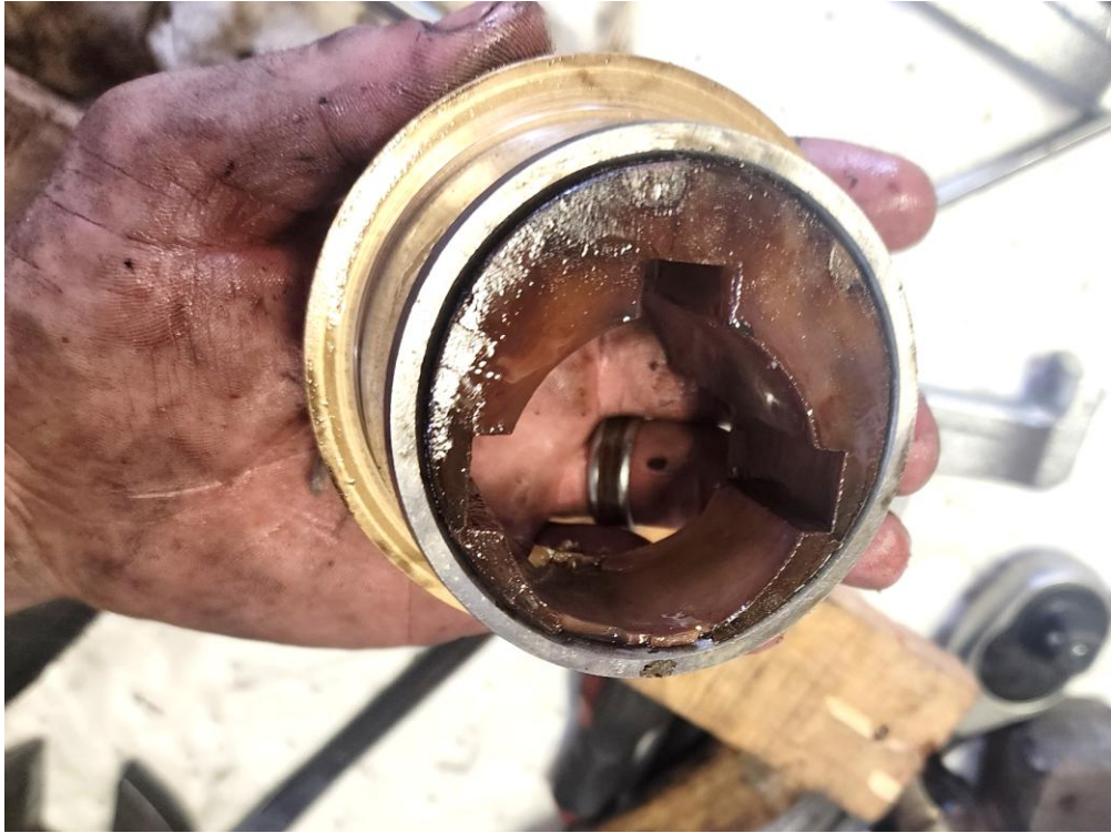
Figure 29: Damage to R1 eccentric (4)
