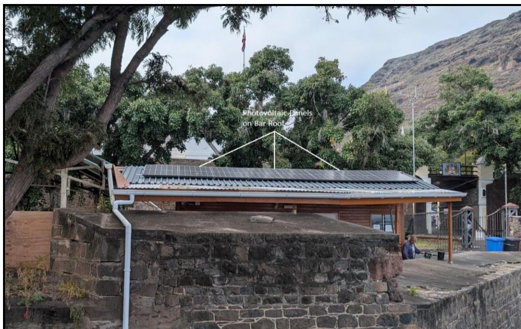
Photograph 1 – Front Elevation Showing Photovoltaic Panels of Bar Roof
