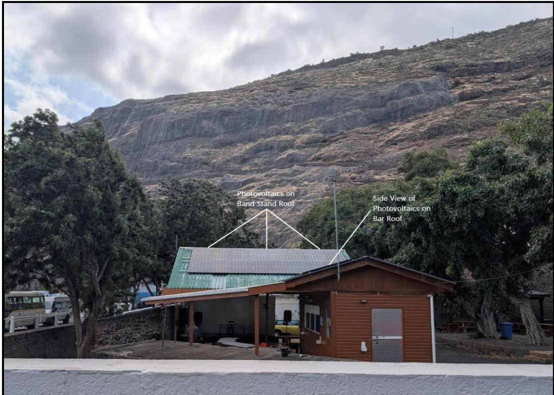
Photograph 2 – West Elevation Showing Photovoltaic Panels on Band Stand Roof and Side View of Photovoltaic Panels on Bar Roof
