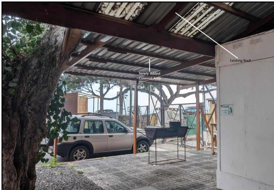
Photograph 2 – Underside of Covered Area Showing Existing & New Roofing
