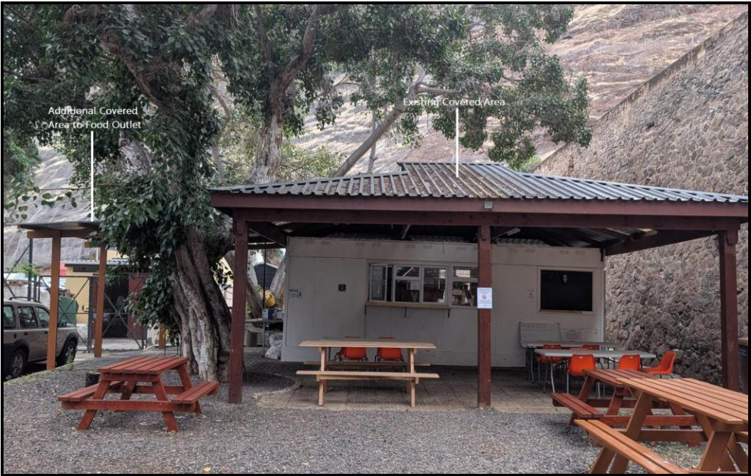
Photograph 1 – Front (West) Elevation
