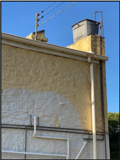
Location of existing water storage tank
