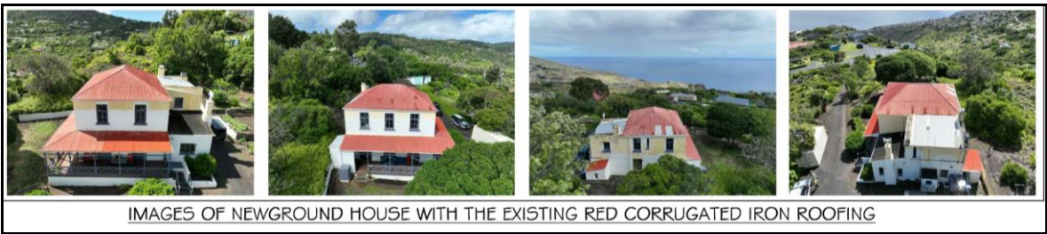
Diagram 3: Photos of existing roof and water tank
