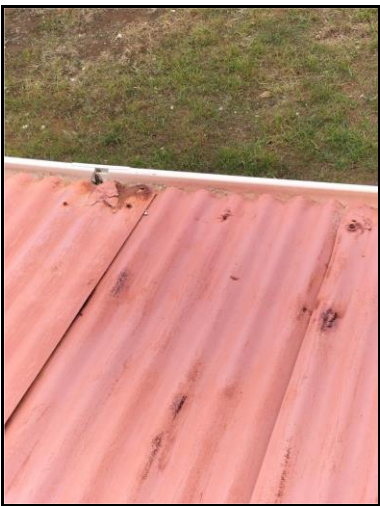
Existing Veranda sheeting condition
