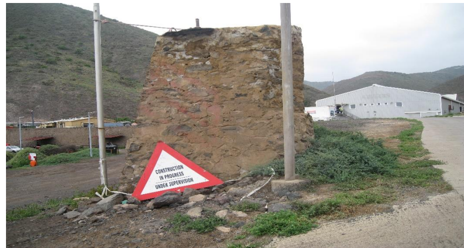
Above – End of the wall showing where previous desecration has occurred.
