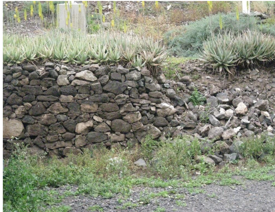
Above – wall to the cliff face
