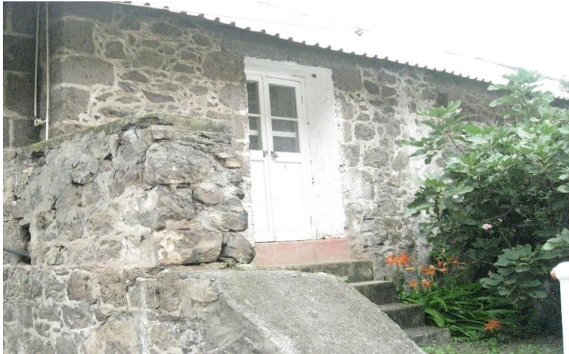
Above – Front of the building
