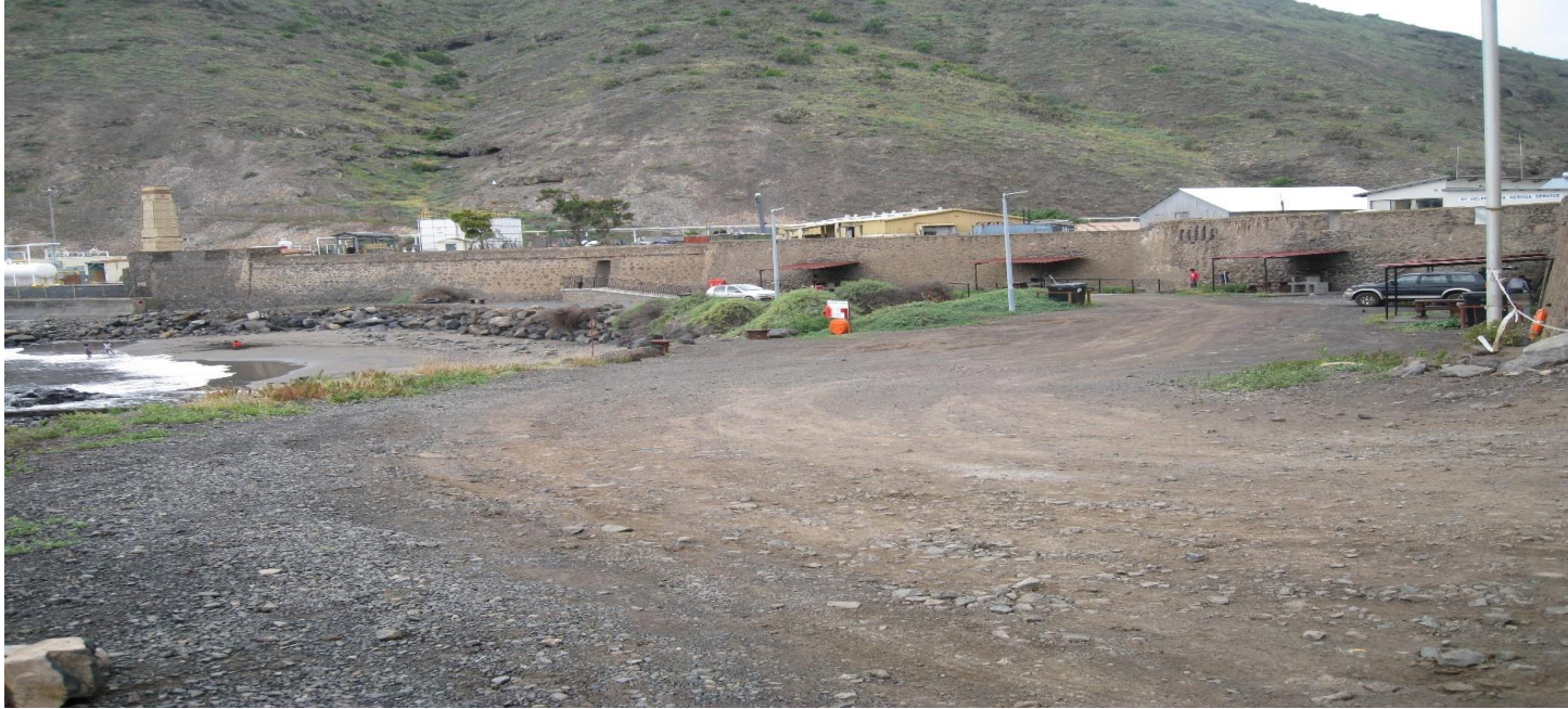
Above – View from the seaward side showing tin shelters erected and pinned to the wall.
