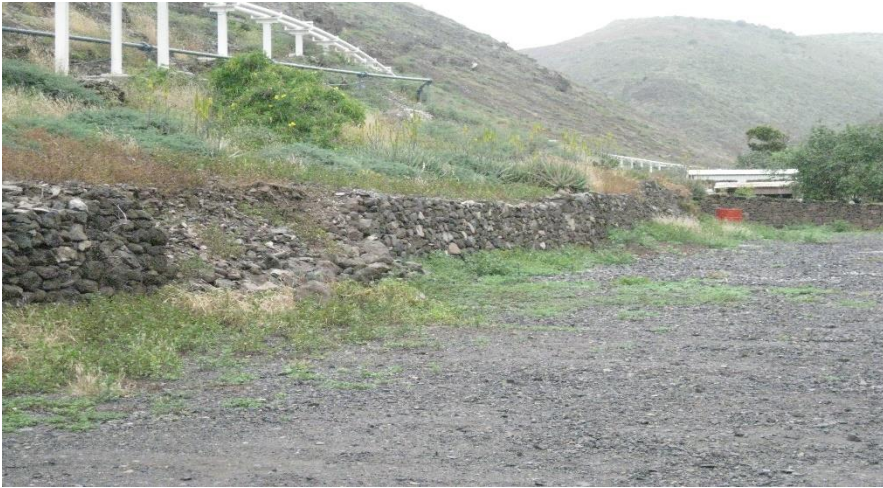
Above – Wall to the cliff face
