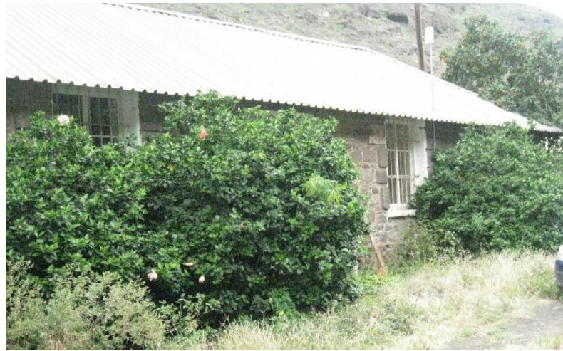
Above – Front of the building
