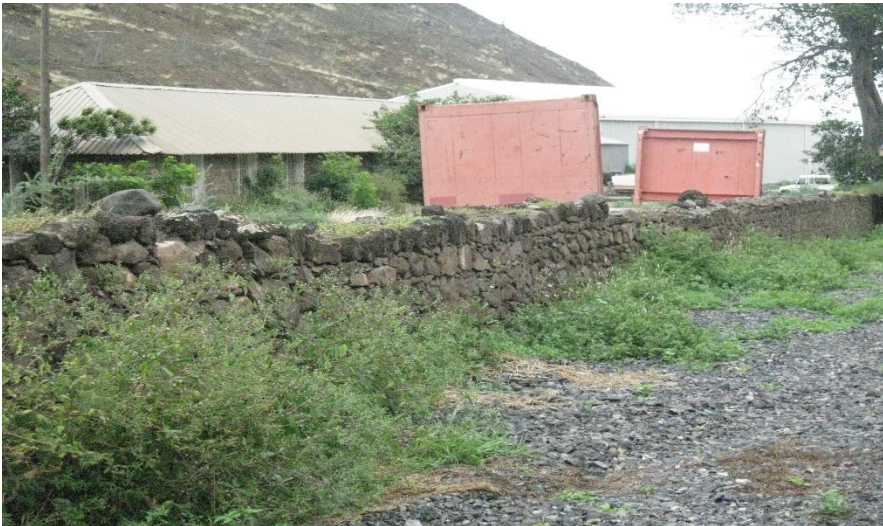
Above – Wall to the main road
