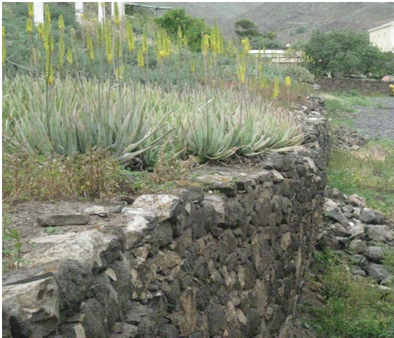
Above – Wall to the cliff face
