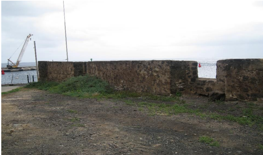
Above – View of the wall with the jetty in the background
