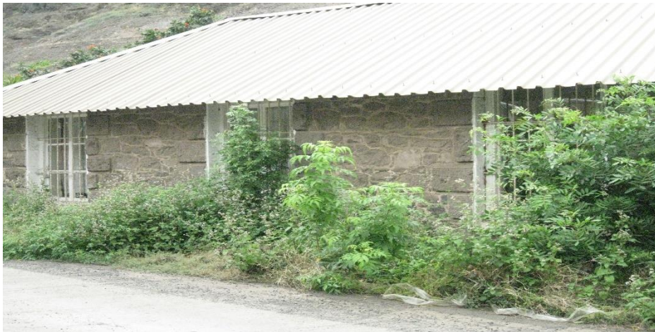
Above – Rear of the building
