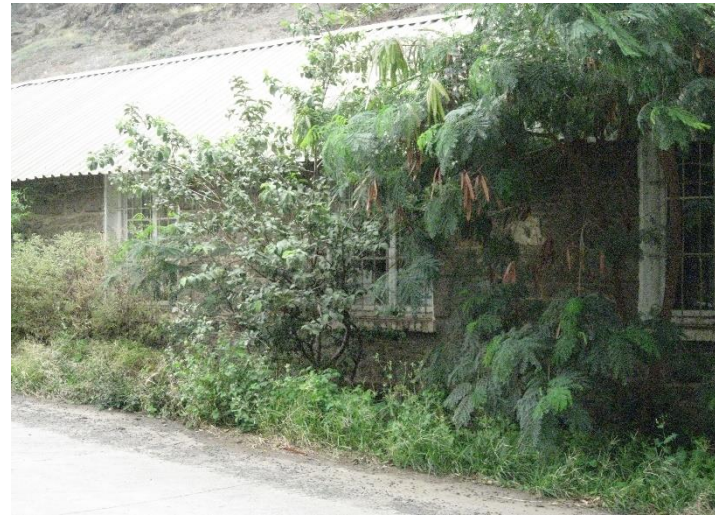
Above – Rear of the building
