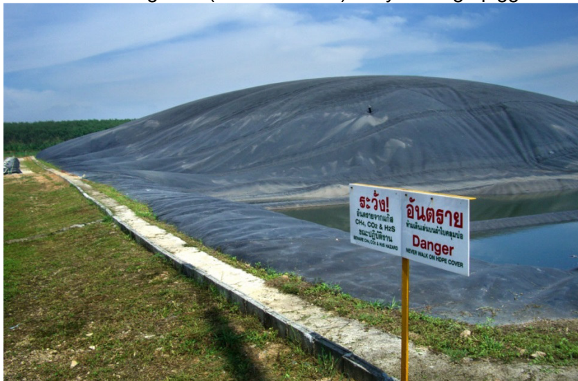
Picture 5: Anaerobic lagoon
