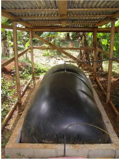
Picture 4: Balloon (sausage) biodigester
