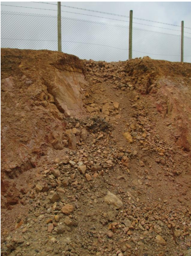
Picture 4; Landslip through erosion at HPLS
