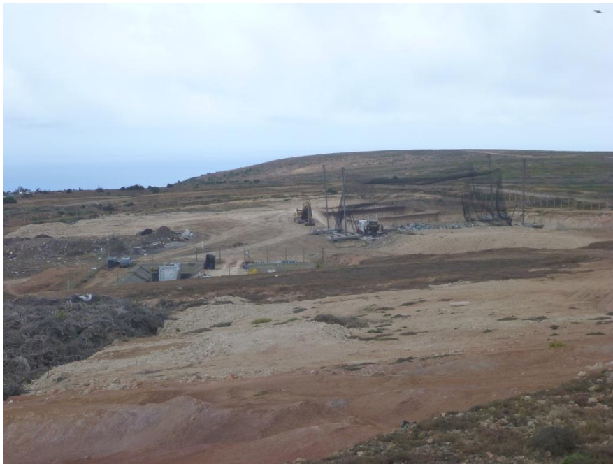
Picture 1; Horse Point Landfill Site (domestic and hazardous waste cells)
