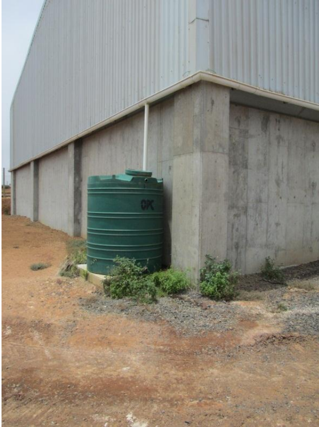
Picture 12 and 13; Rain water collection tanks fitted to either end of the Waste Reception Building
