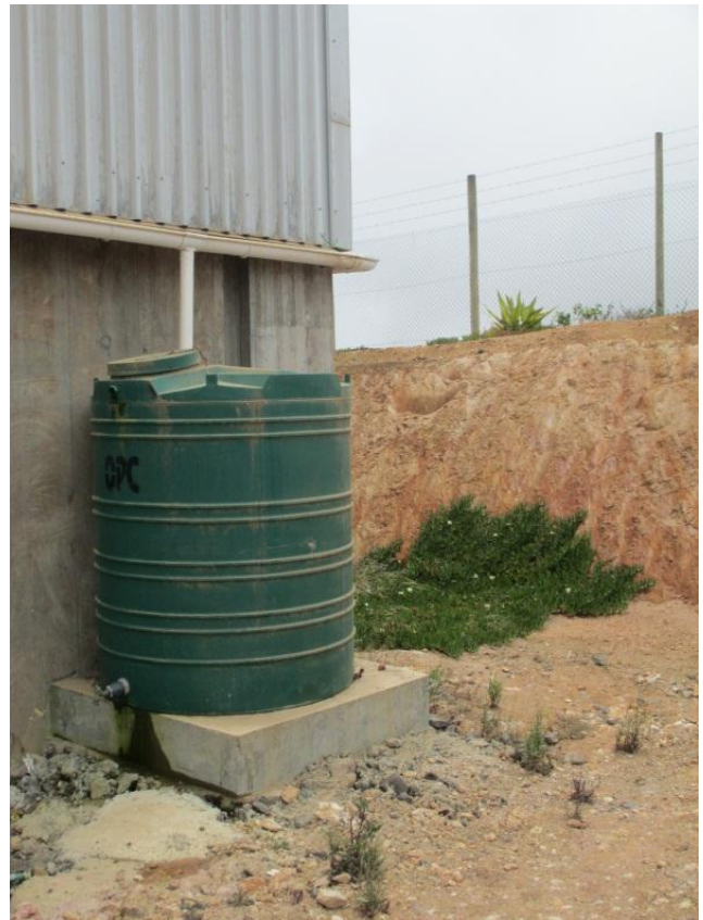
Picture 12 and 13; Rain water collection tanks fitted to either end of the Waste Reception Building
