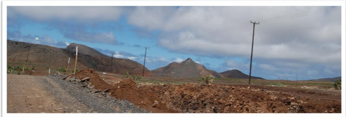
Fig 5. Photo looking towards Tungi Flats showing the continuation of the electricity lines down to the area of the batch plant. (Travelling from Airport Site)
