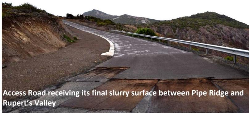
Access Road receiving its final slurry surface between Pipe Ridge and Rupert's Valley
