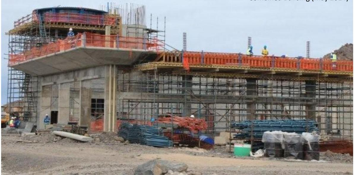
The Airport buildings at Prosperous Bay Plain are now well advanced. The structure of the Combined Building which will house Air Traffic Control and Rescue and Fire Fighting Services is now 79% complete. Brickwork is 74% complete and plastering 9% complete. The Control Tower structure is also in place and the steel structure of the control room is being painted prior to erection.
