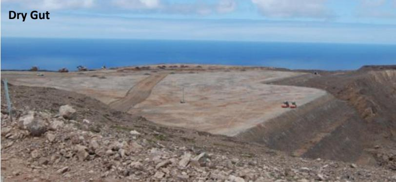
Earlier this month the Dry Gut fill reached 270m in height. The filling of Dry Gut is required to extend the platform available for construction of the runway and the runway end safety areas.
