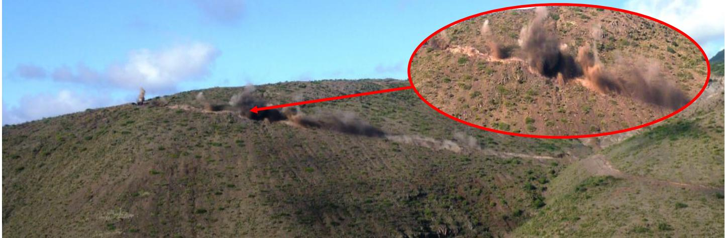
Blasting on the Haul Road in upper Rupert's Valley took place on Tuesday 11 March 2014 just after 5pm. The main purpose of the blast was to assist the heavy plant to excavate the harder section of the track to improve the widths and the gradients to form an Access Road for ultimate public use in the future. 8,513kg of high energy fuel (explosives) was used in the blast - it lasted 5.78 seconds and produced 17,881m<sup>3</sup> (approx 34,000 tonnes) of material.
