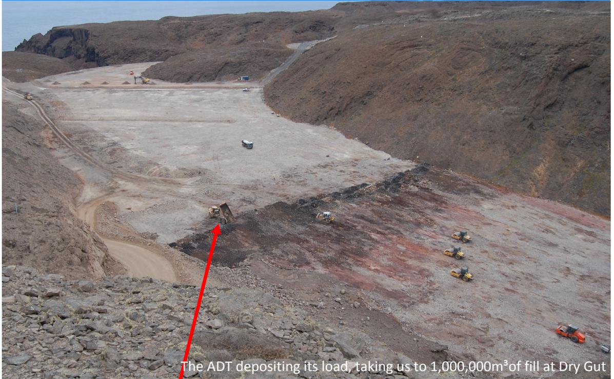
The ADT depositing its load, taking us to 1,000,000m<sup>3</sup> of fill at Dry Gut
