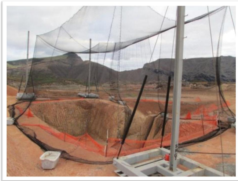
Figure 3.1: First waste cell cut at HPLS prior to filling August 2014
