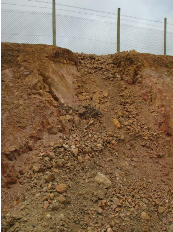
Picture 1; Landslip through erosion at HPLS
