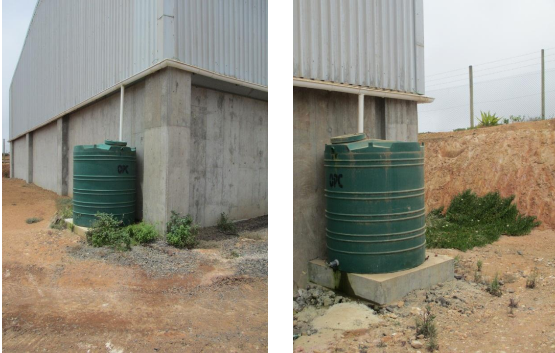
Picture 9 and 10; Rain water collection tanks fitted to either end of the Waste Reception Building
