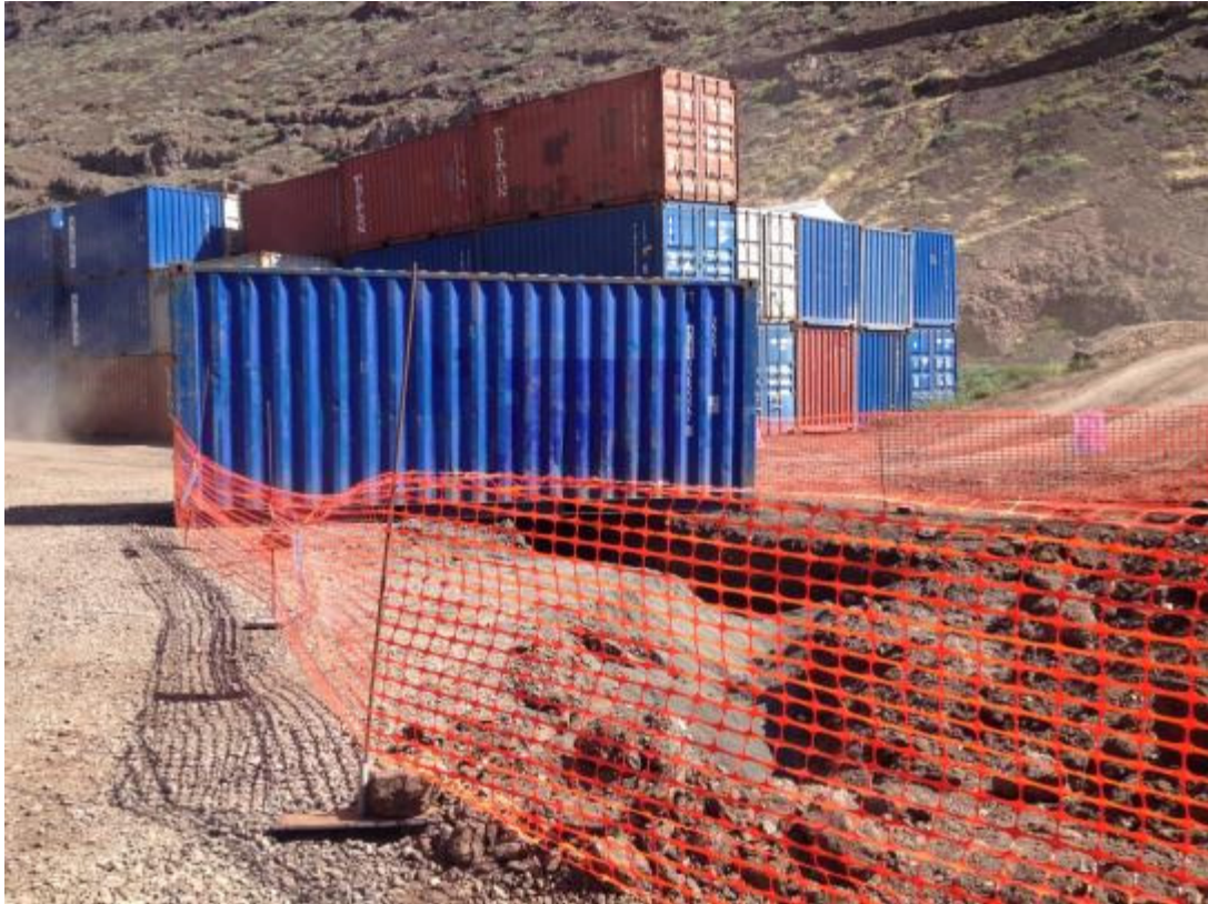
Plate 4: Temporary Backfill of Excavation and Barrier
