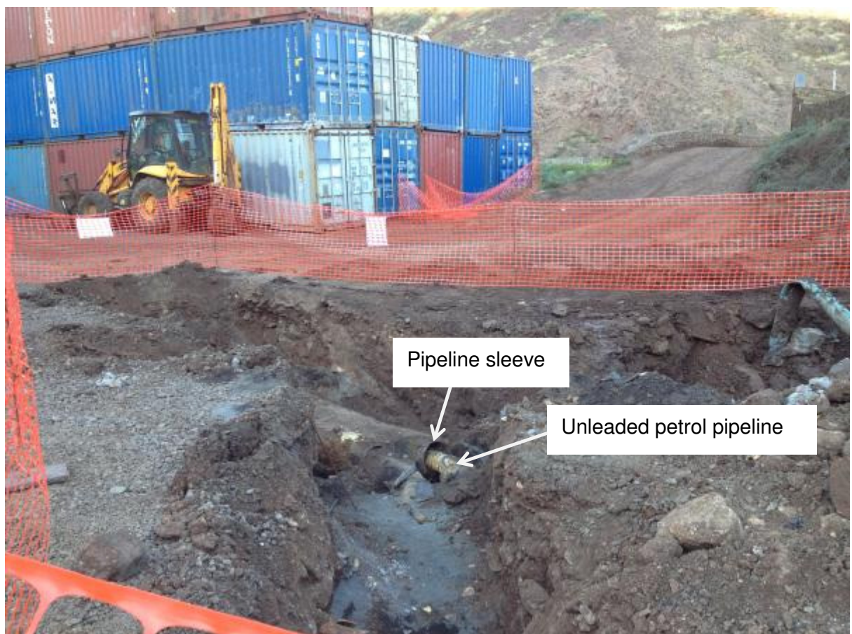
Plate 1: Exposed pipe, sleeve and excavation
