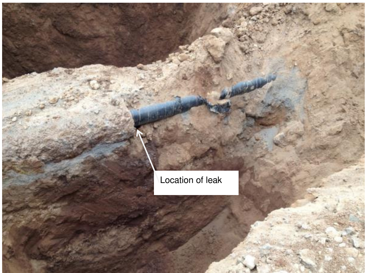
Plate 5: Location of Leak in Unleaded Petrol Pipeline
