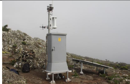
Plate 17: One of the remote obstacle lights on top of The Barn. Note solar panel on the right.
