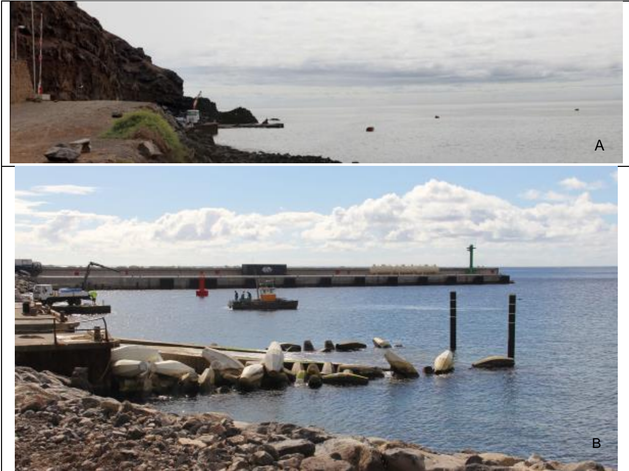
Plate 44: Rupert's Bay prior to the construction of the permanent wharf in April 2013 (A) and after completion in June 2016 (B)
