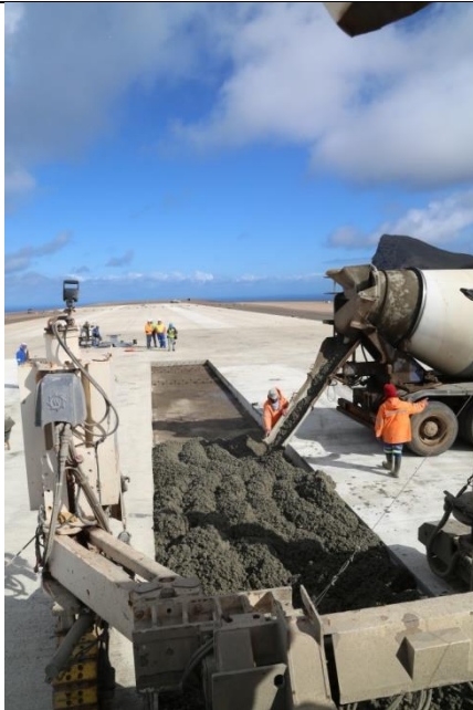
Plate 14: Pouring the last concrete on the airport runway
