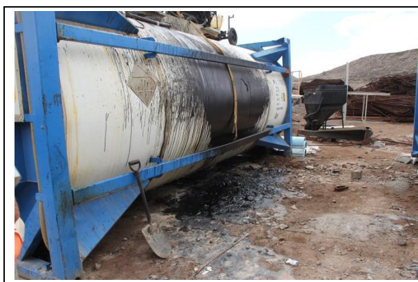
Plate 9: Poor bitumen management was observed in several places during the February 2016 audit
