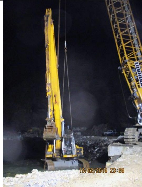
Plate 6: An excavator fell into the sea at the permanent wharf. Oil spill protection was deployed immediately as per CEMP
