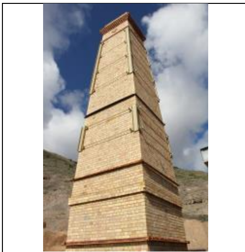
Plate 38: Desalination chimney with bracing in place
