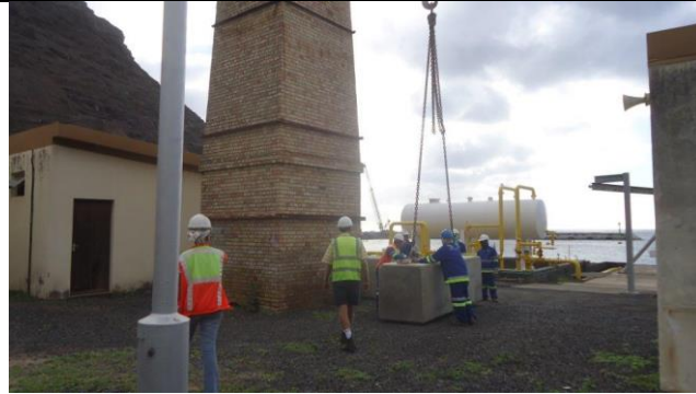
Plate 37: Placing the concrete barriers around the base of the chimney under the supervision of Gideon Niemand and Annina van Neel
