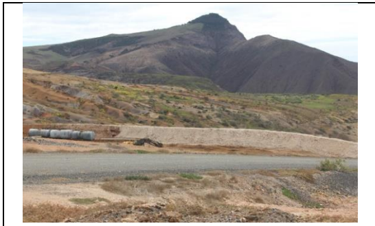
Plate 39: The new bulky waste cell at Horse Point landfill site constructed by BR for joint use by BR and EMD. (Note that the tanks were being stored here on a temporary basis)
