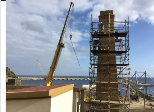
Plate 36: Installation of the protective braces on the chimney
