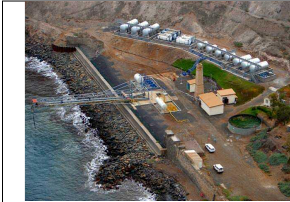
Plate 30: Aerial view of the Bayside BFI prior to demolition
