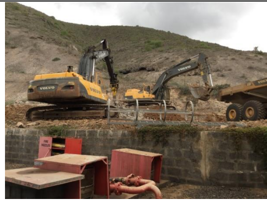
Plate 31: Excavators at work removing the tank platform to make way for the new BFI
