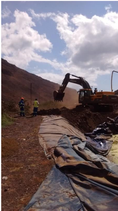
Plate 5: Scattered human bones were found during removal of the temporary reservoir in Rupert's Valley. Work stopped immediately as per CEMP
