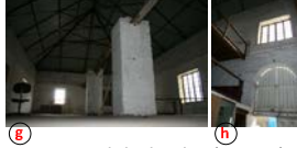
PWD store existing interior photographs
