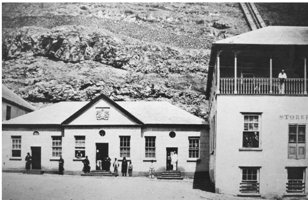
A complex of three linked and interlinked buildings fronting the Grand Parade
