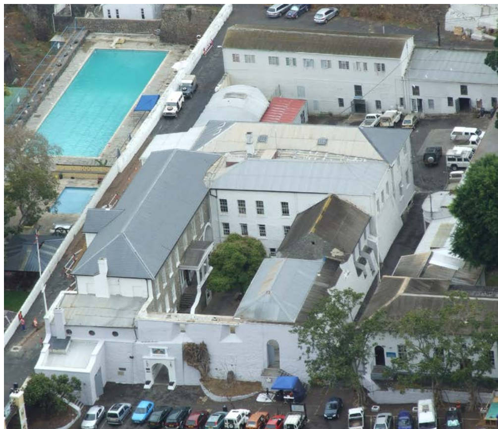
The Castle and rear PWD Yard area as viewed from Ladder Hill.
