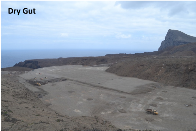
Levelling of the Platform for the Combined Building
