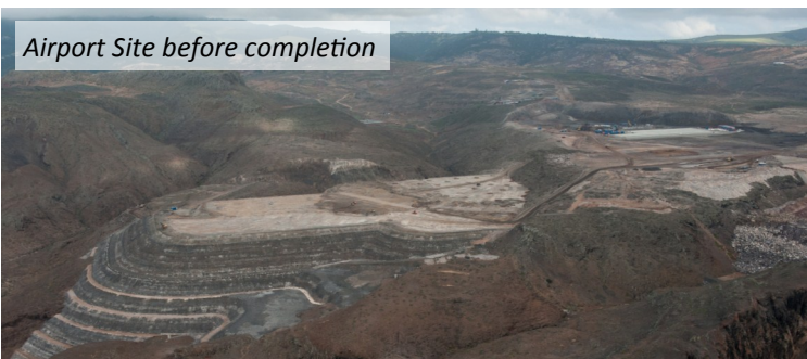
St Helena Airport
